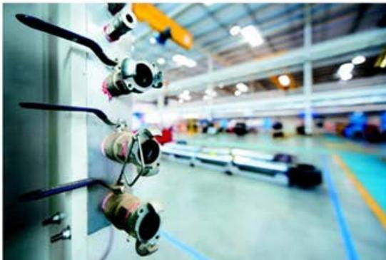
With seven manifold outlets installed at different points throughout the facility, compressed air is highly accessible when and where required.
